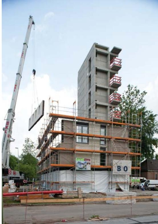
Figure 8: Holz8 building employed pre-cast concrete for the cores, contributing to a very quick construction time of 16 days (Architecture by: Schankula Architekten, Photo credit: Huber & Sohn).
