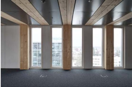
Figure 7: Ceiling panels between timber beams conceal systems at LCT ONE (Photo Credit: www.creebuildings.com).
